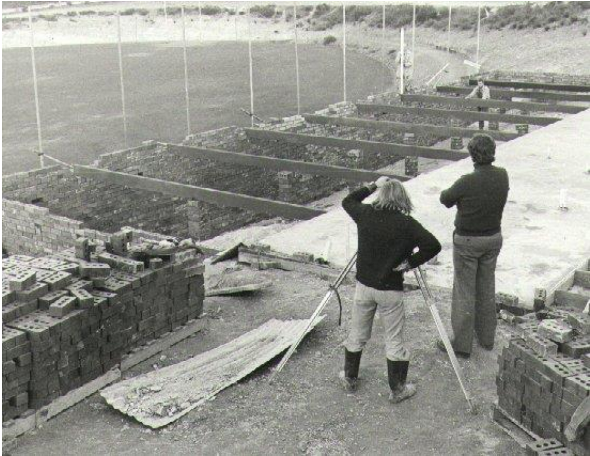
Checking the levels on the new clubrooms.
