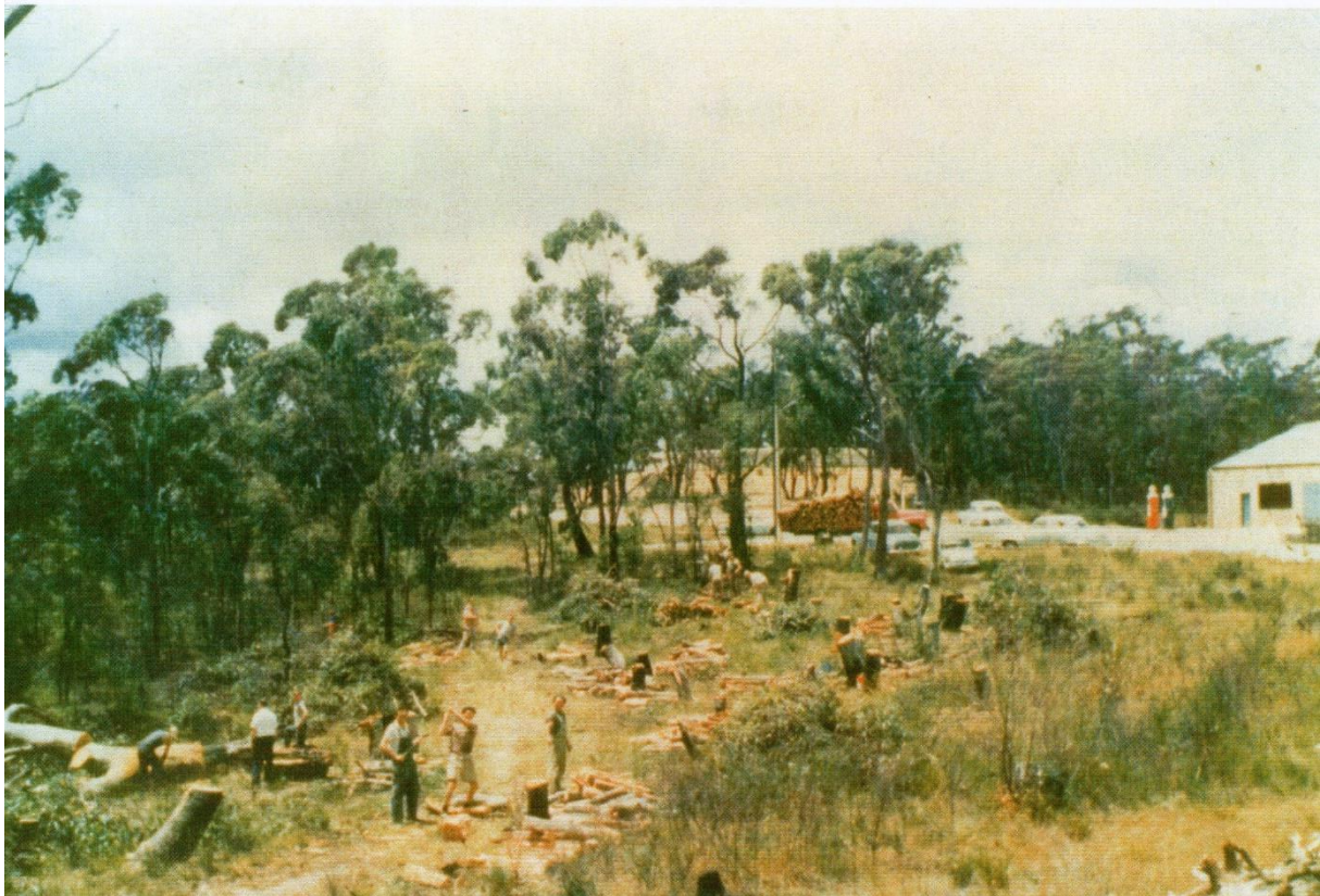
In early 1963 work has commenced to create the new oval
