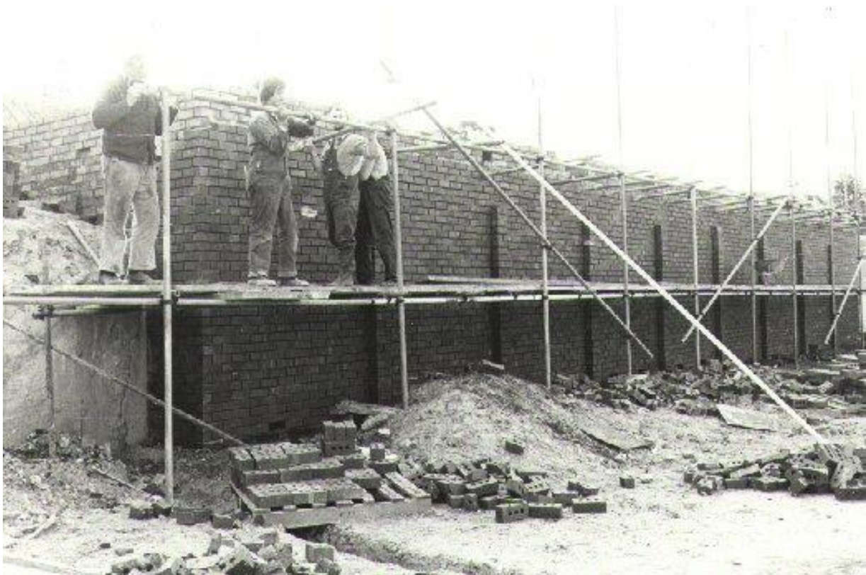
Construction of Stage 1 is underway.
